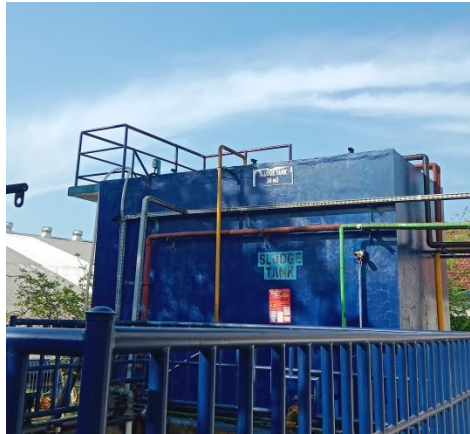
Gambar 4. 11 Sludge Tank (Sumber : PT Tirta Investama (AQUA ) Pandaan)
