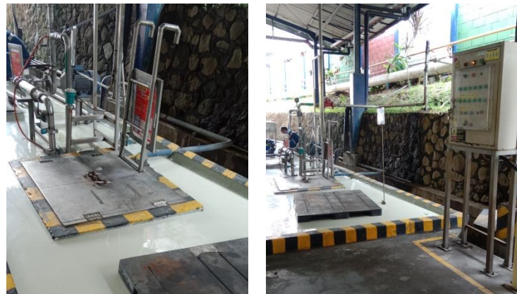
Gambar 4. 5 Pumpit (Penampung Limbah Beverage Mizone) (Sumber : PT Tirta Investama (AQUA ) Pandaan)
